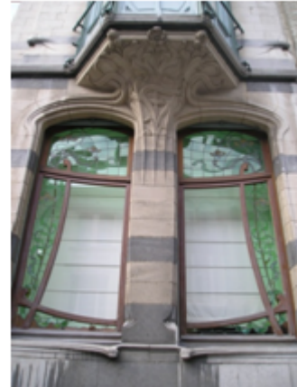
Figure 1: A Similar Window Detail in Brussels, Belgium
